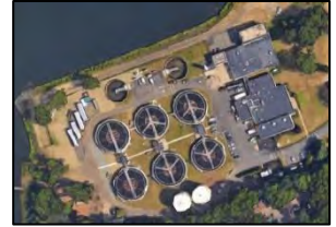
E – Central Swimming River Filter Plant
