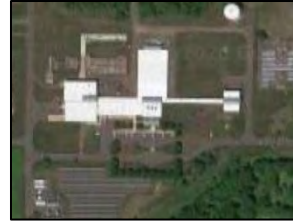
D – Central Canal Road Water Plant
